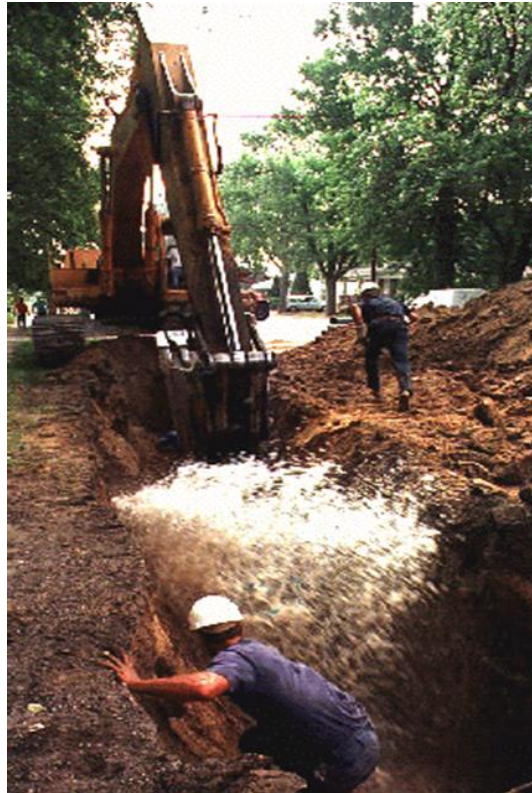
Workers escaping deep trench after a backhoe has burst a water main. While most trench fatalities are from cave-ins, drownings, electrocutions, asphyxiation and explosions are additional risks associated with water, sewer, gas and electric lines.
