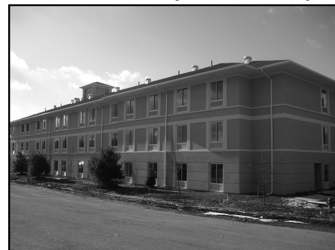
Hotel constructed using ICFs
