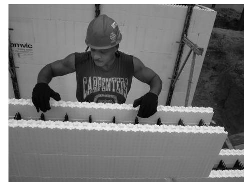
Union Carpenter installing ICFs
